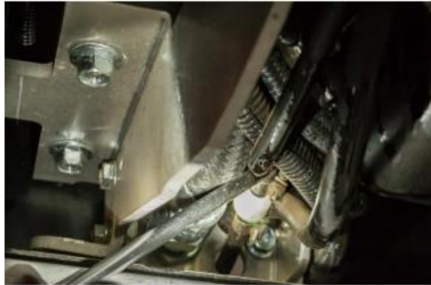
Fig 19b (Valve seen from beneath the unit)
