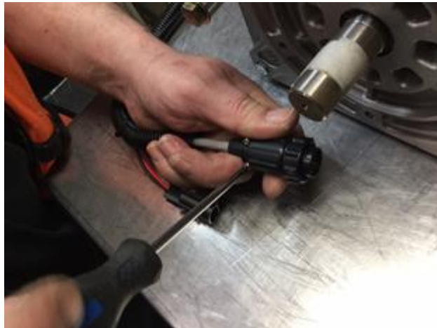
Figure 4 – Plug disassembly
