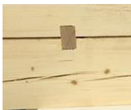
Figure 10. Timber infill for shear force
