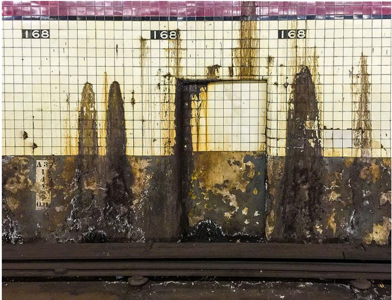
A subway station at 168th Street in Manhattan (Wikimedia)
