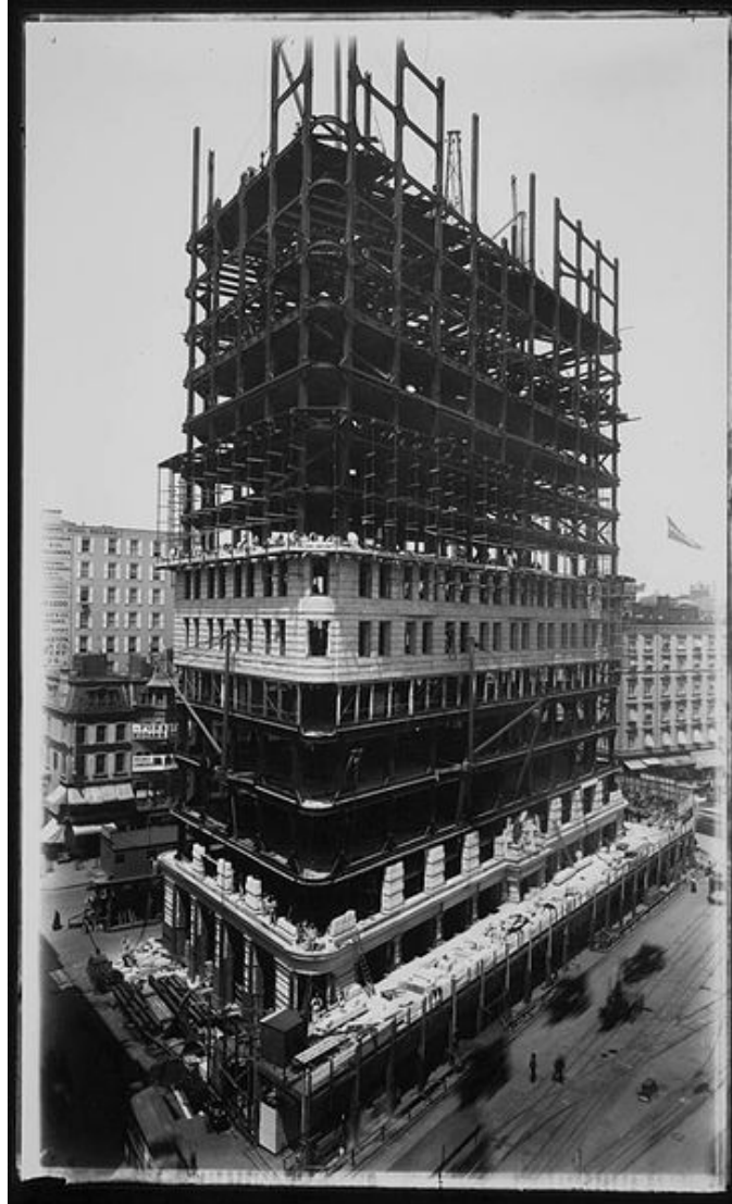
Construction of the Flatiron Building, New York City, ca. 1905 (Wikimedia)
