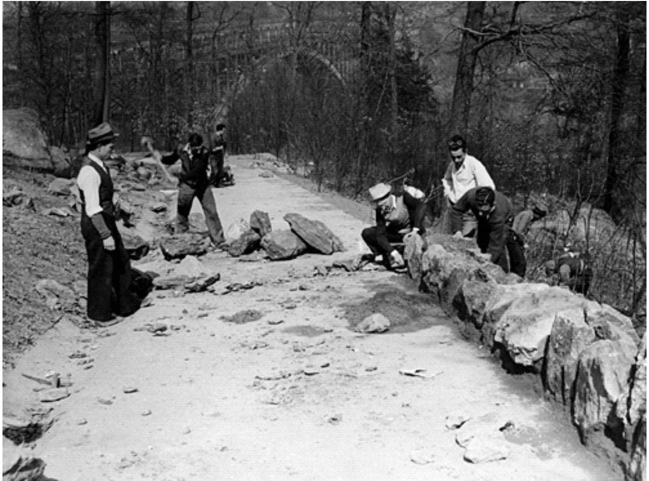
WPA workers, in 1938, constructing a paved pathway in Inwood Hill Park (The Works Progress Administration)
