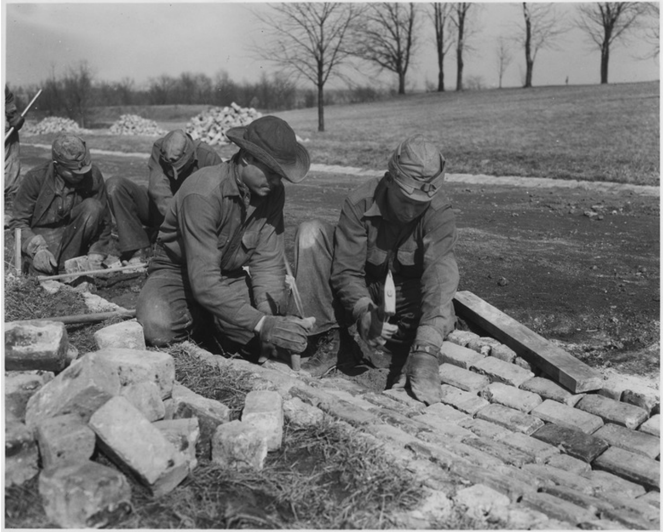
Members of the Civilian Conservation Corps (CCC) laying bricks (Wikimedia)
