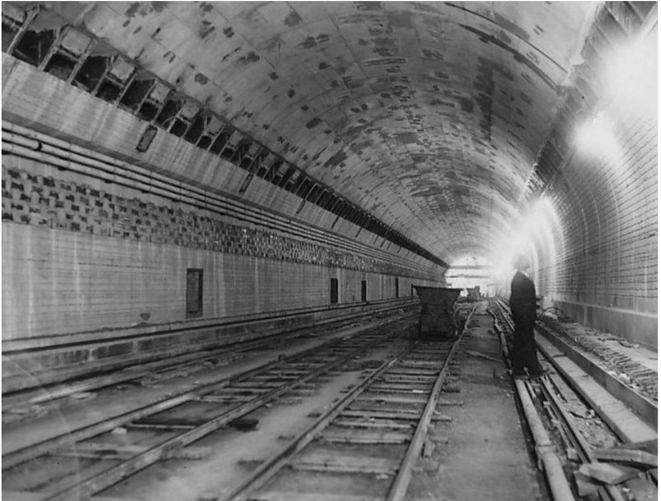
The Lincoln Tunnel in New York City connects lower Manhattan to New Jersey. The tunnel, built thanks to the Public Works Authority from 1934 to 1937, remains an essential commuter tunnel in New York today. (Wikimedia)
