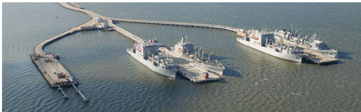
The Naval Weapons Station Earle Pier Complex supplies the Carrier and Expeditionary Strike Groups in the Atlantic. The three-mile-long pier allows ammunition trains to quickly and safely load USNS auxiliary ships supplying the Fleet. Navy photo by Naval Weapons Station Earle.
