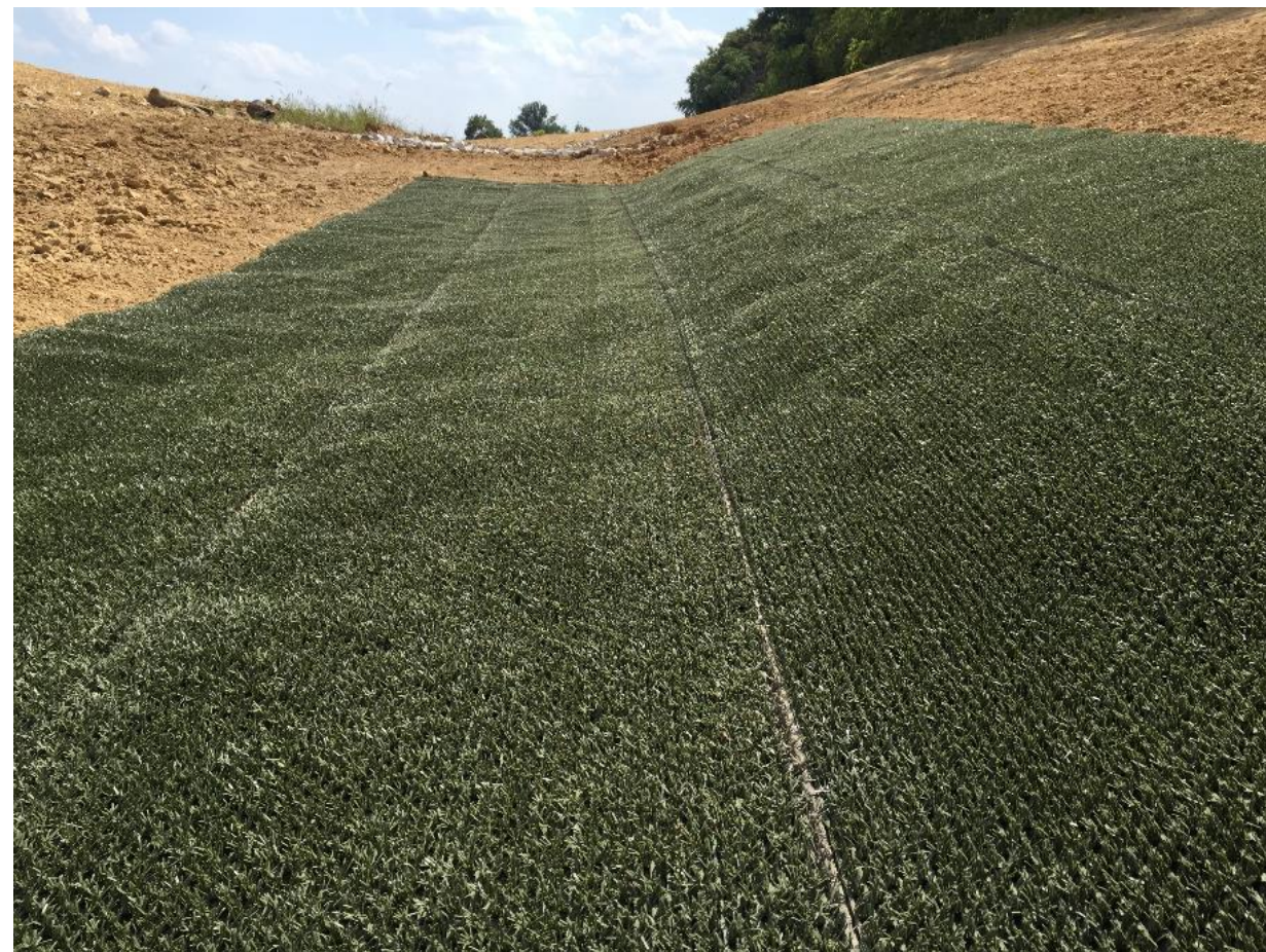
Upslope view of ShearForce10 just after installation on Sep 10 (left) and on Nov 20 (right).
