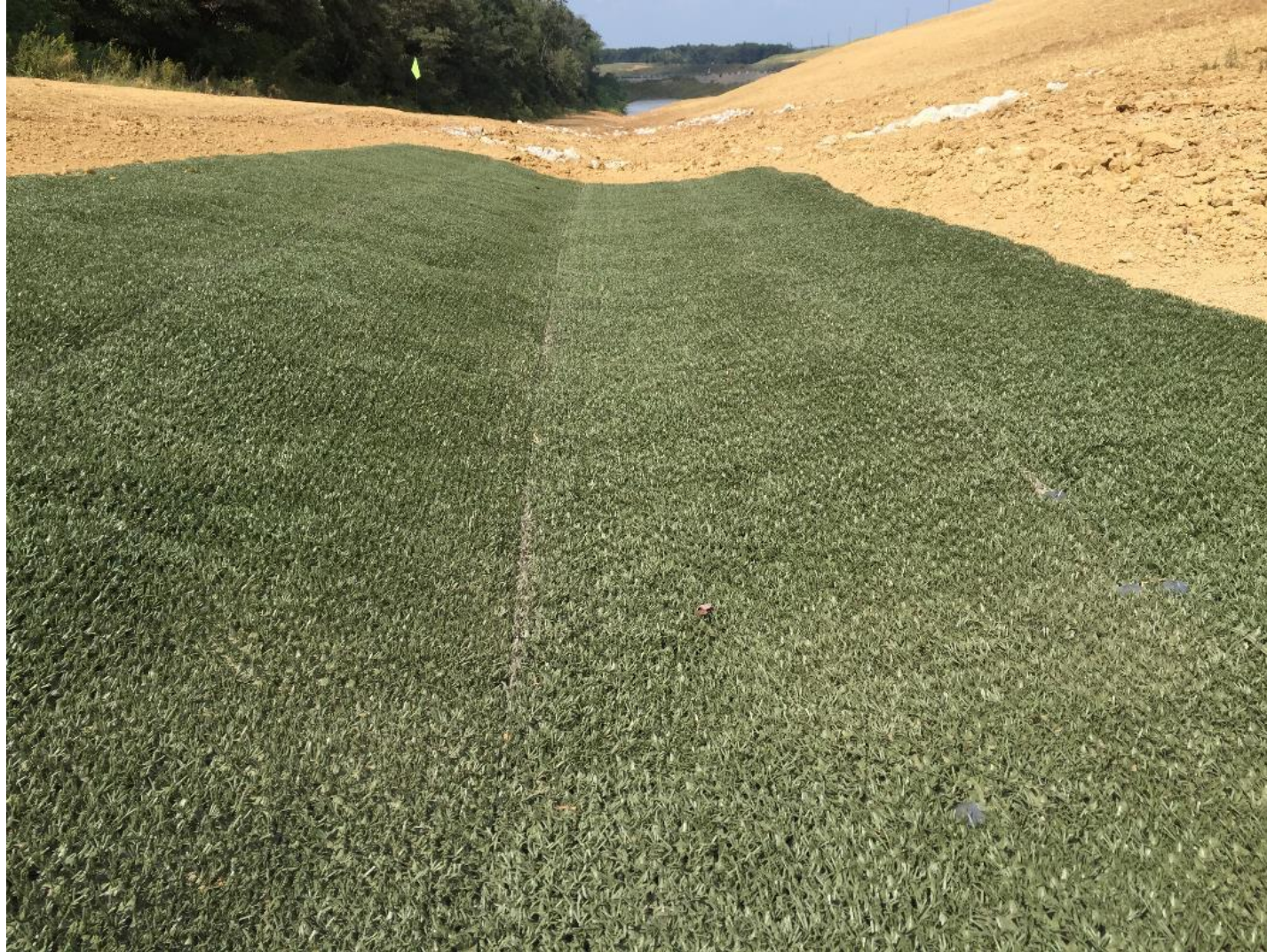
Completed ShearForce10 Installation looking down channel grade
