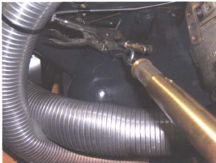
Figure 2. Scale pulling in line with cable.
