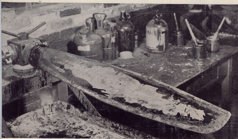
6—(Above) With the blade covered with the plastic sheet, it is left to cure after which overlap is cemented flat on the thrust face. 7—(Below) Sanding of the cured blade is accomplished after the lap joint has been cut off. Templates are used to check uniformity
