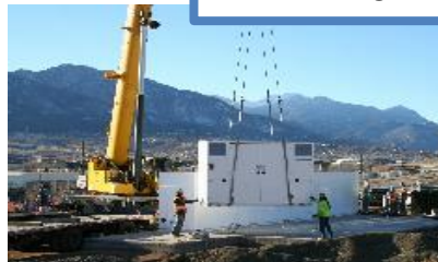
Fort Carson, CO: A 4.2 MW / 8.5 MWh battery energy storage system that is the largest peak-shaving battery on an Army installation and will offset peak electric use to reduce installation energy costs.
