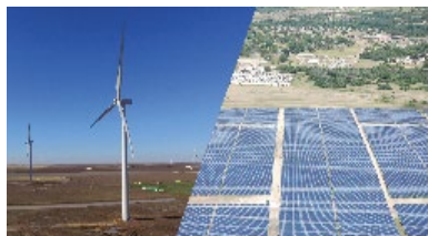
Fort Hood, TX: The Army's first hybrid solar and wind energy Power Purchase Agreement has a capacity of approximately 65 MW AC, enough to power about 21,000 homes.
