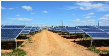
Fort Detrick, MD: A 15 MW Solar Facility comprised of 59,994 Solar Panels that generates enough electricity to power about 2,720 homes.
