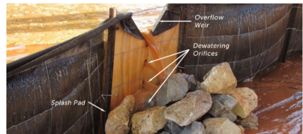
Fig. 1: Example dewatering board & overflow weir.
