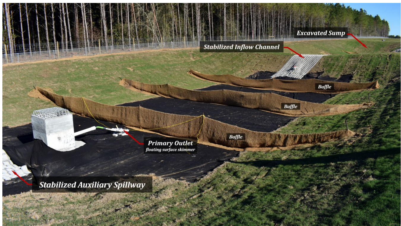
Figure 1. Example sediment basin design elements.
