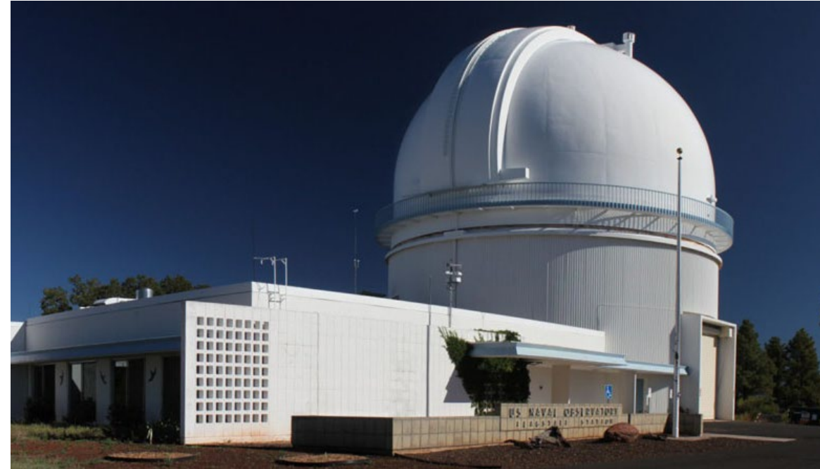
Main building of the USNO Flagstaff Station, (NOFS) in Flagstaff, Arizona (U.S. Navy Photo by Geoff Chester)
