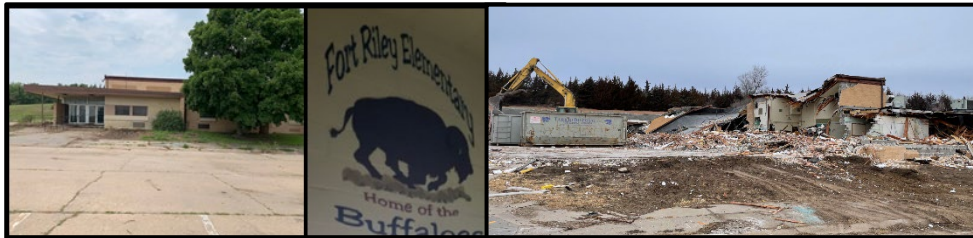
Old Fort Riley Elementary School Demolition
