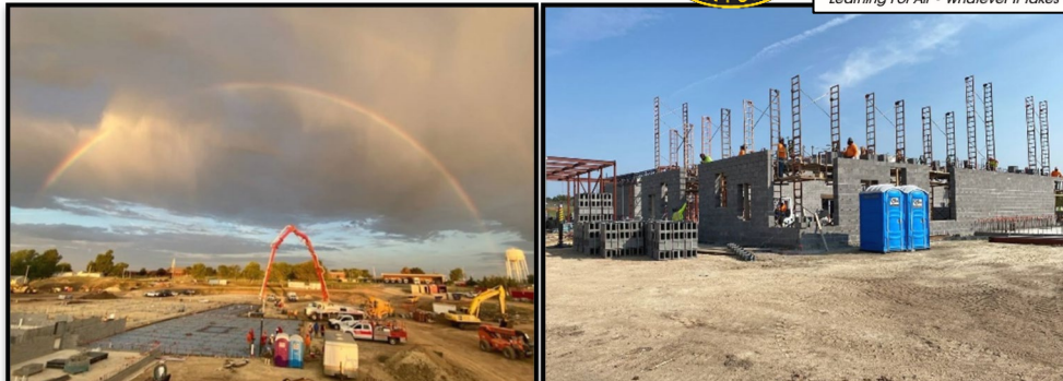
New Elementary School Construction on Fort Riley
