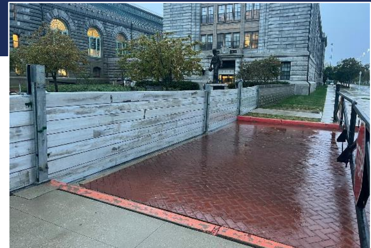
Deployable Flood Barrier across Roadway
