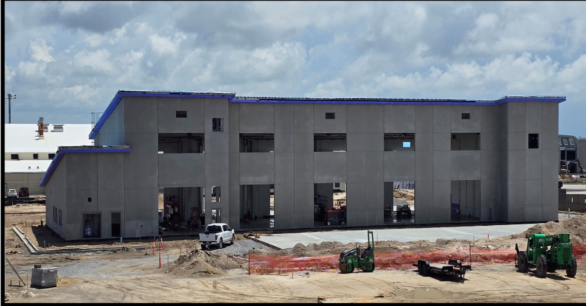
FIRE TRUCK / MATERIAL HANDLING EQUIPMENT MAINTENANCE FACILITY
