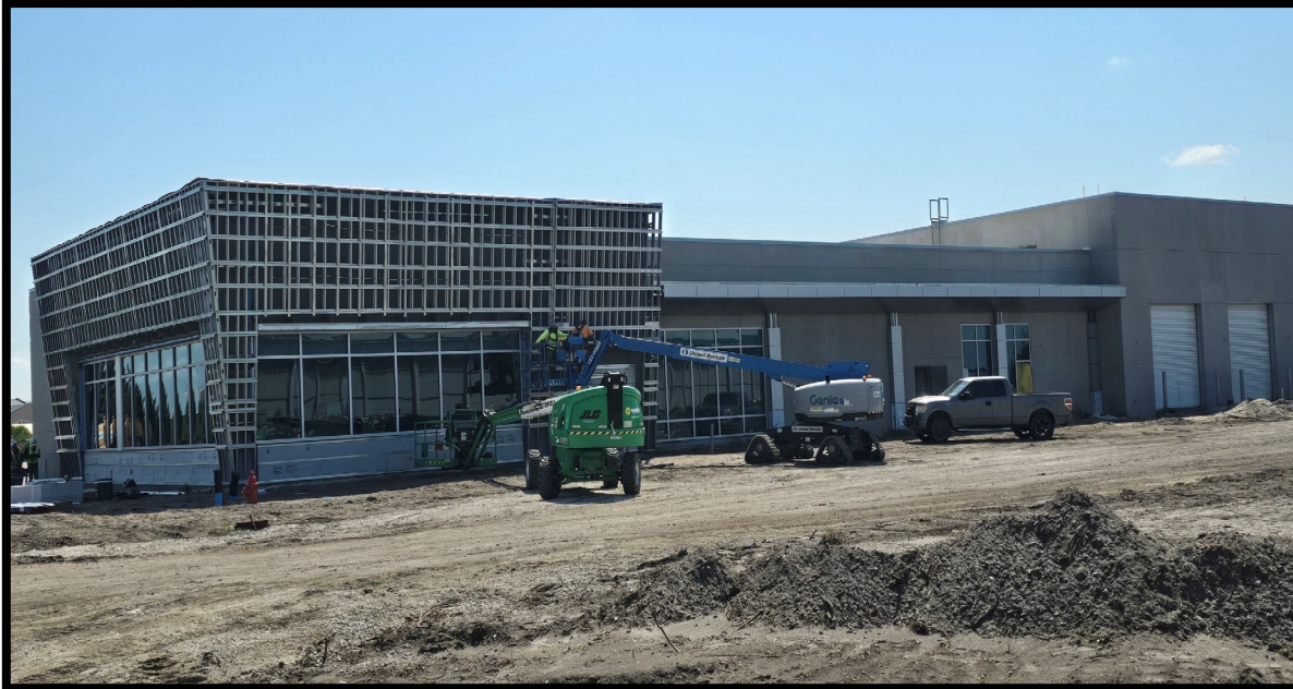
EXPLOSIVE ORDNANCE DISPOSAL FACILITY
