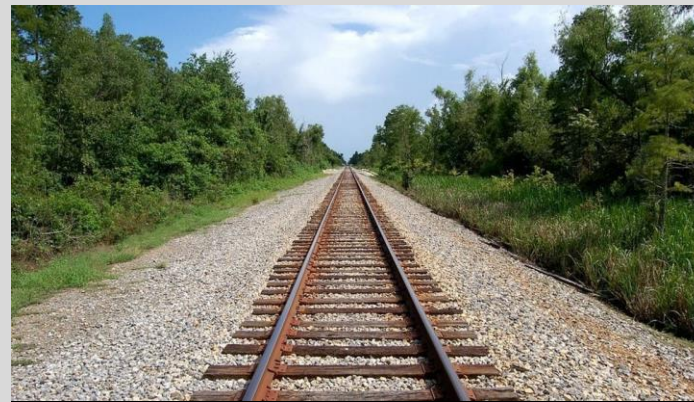
New Railroad Tracks
